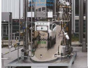
reliable centralised gas supply solution for small cryogenic storage tanks. For customers whose gas consumption exceeds the gas supply from cylinders, the Microbulk ensures a more reliable and hassle free supply. This gas supply solution is designed for outdoor installations and comes with various storage capacities suited to the different customers needs.
